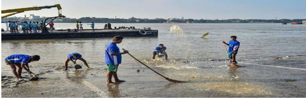
WORK UNDER NAMAMI GANGE PROJECT IN UTTAR PRADESH.
